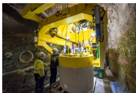
Fig. 6 Buffer installation demonstration in Onkalo URFC.
