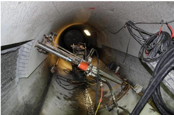
Instrumentation drilling of sensor holes, the sawed out cable notches can be seen on the drift sides
