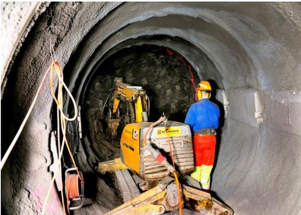
Excavation of experiment tunnel with a pneumatic hammer
