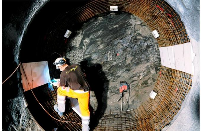
Tunnel support made with steel nets and shotcrete
